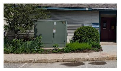
Figure 15 6 Spruce St. Electrical Distribution Transformer
