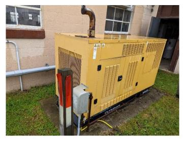
Figure 11 Existing Diesel Generator Providing Lighting Power to Motor Pool During Outages
